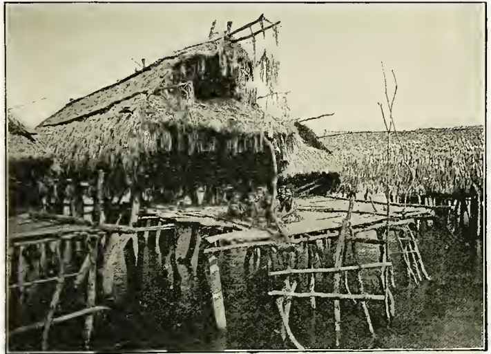
FIG. 307. — A village in New Guinea, where the houses are built on posts rising above the water.
